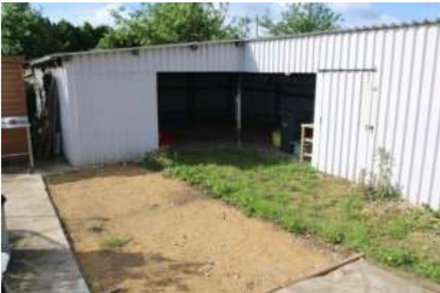
Concrete floor done, old roof cladding removed and new roof timbers where needed. Many of the old timbers were warped, rotten or in the wrong place. Additional beams were required to provide the correct spacing for the new roof cladding.
